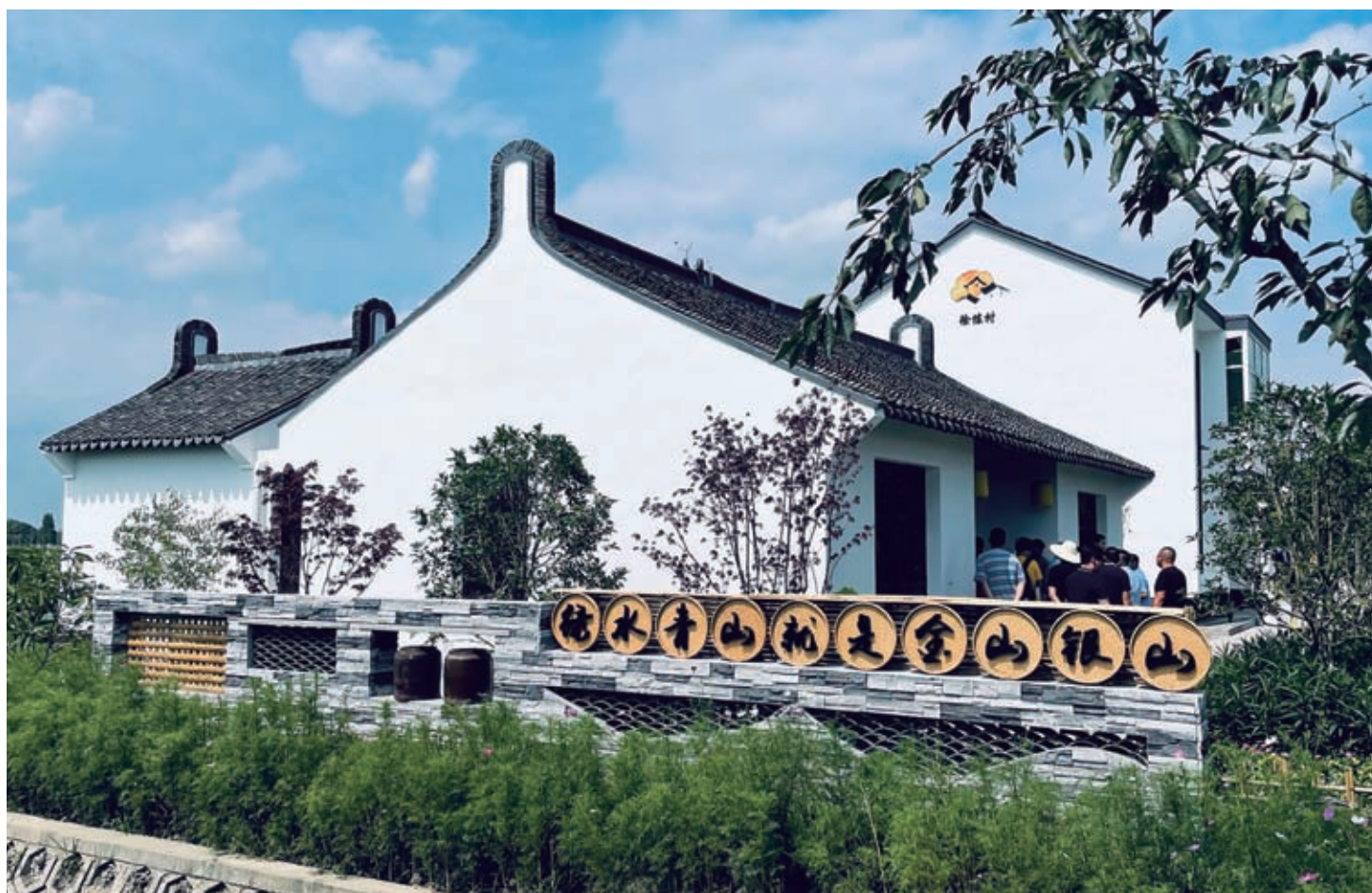
The balancing act of rural architects is to improve local lifestyles without doing harm to the natural environment. — Ti Gong
